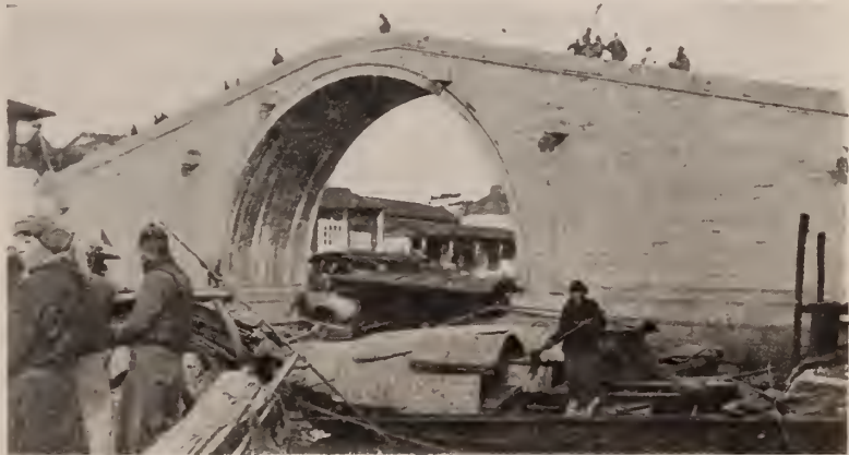
Bridge over the Canal which encircles the City of Soochow.
